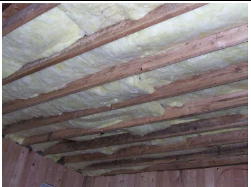
Insulation before the vapor barrier
