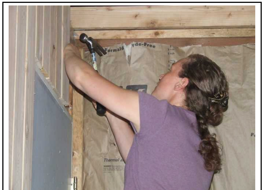
Debbie installing siding over the back door
