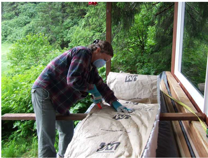
Debbie cutting insulation on the porch
