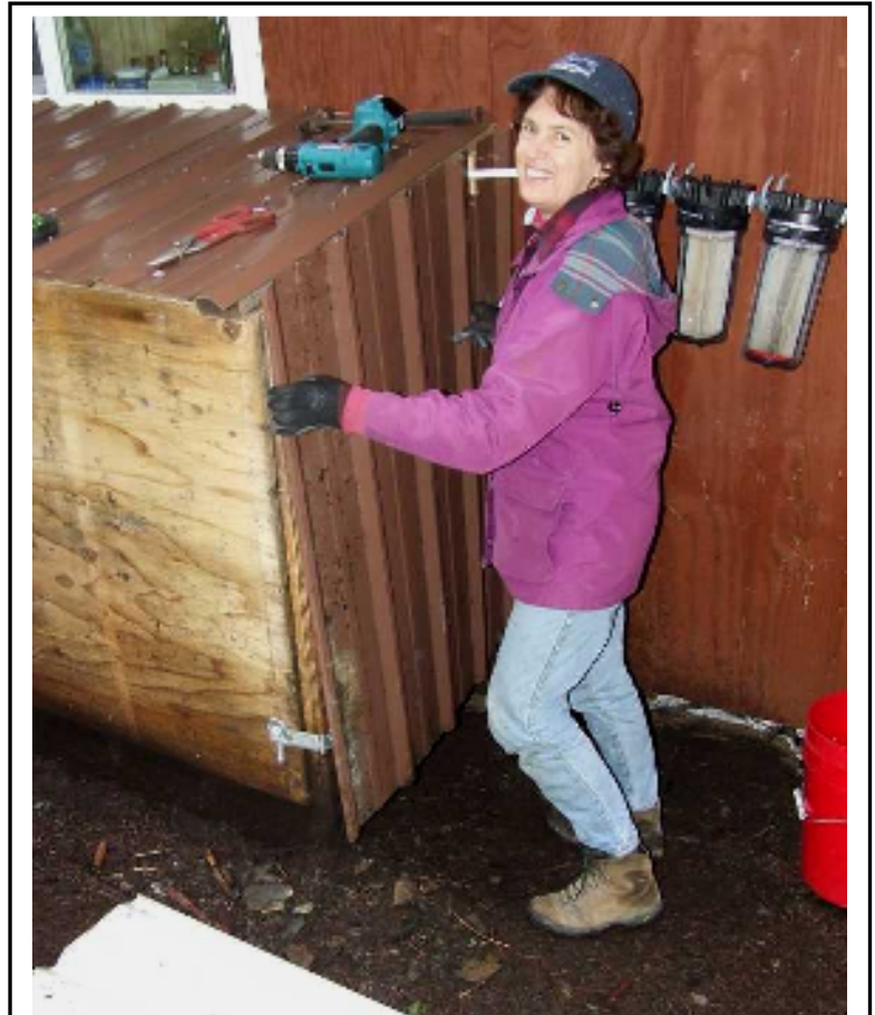
Mom putting up metal roofing on the bear proof box
