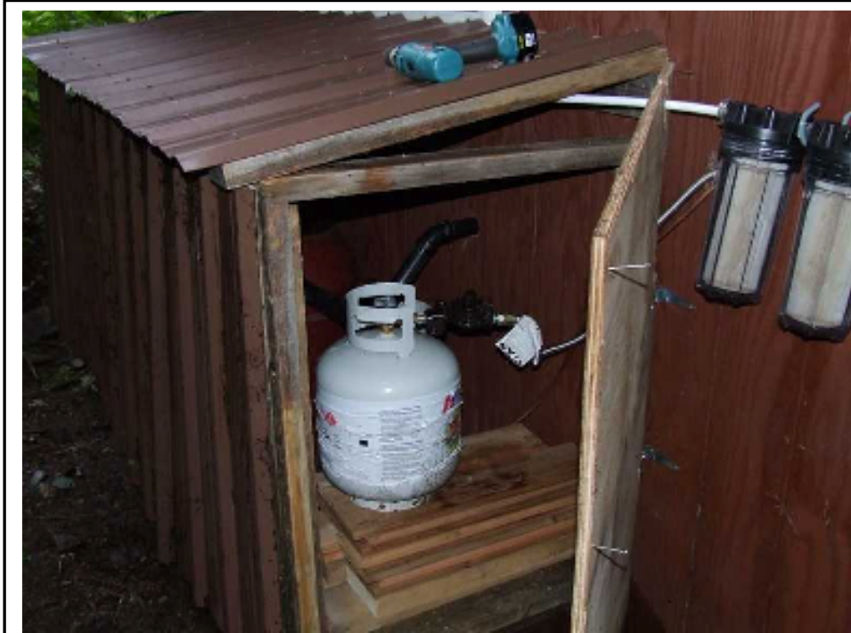
One end of the bear proof box with metal roofing and propane tanks inside
