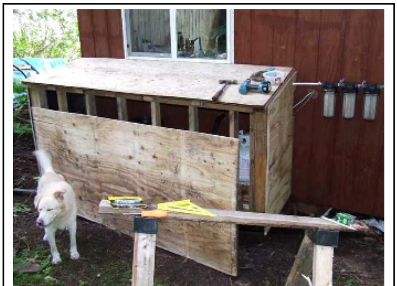
The bear proof box under construction
