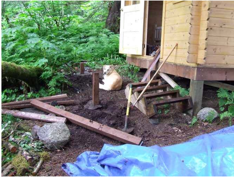
Constructing Cottonwood Cabin's porch
