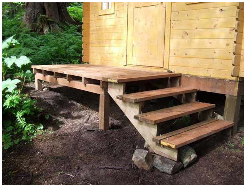
The finished porch
