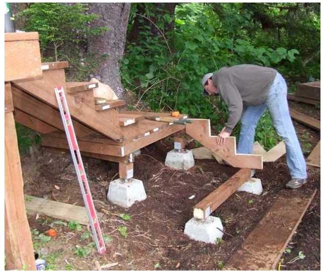
Carp finishing the stairs
