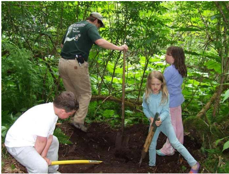
Glenn, Allison, Hope and Steven working on the outhouse hole
