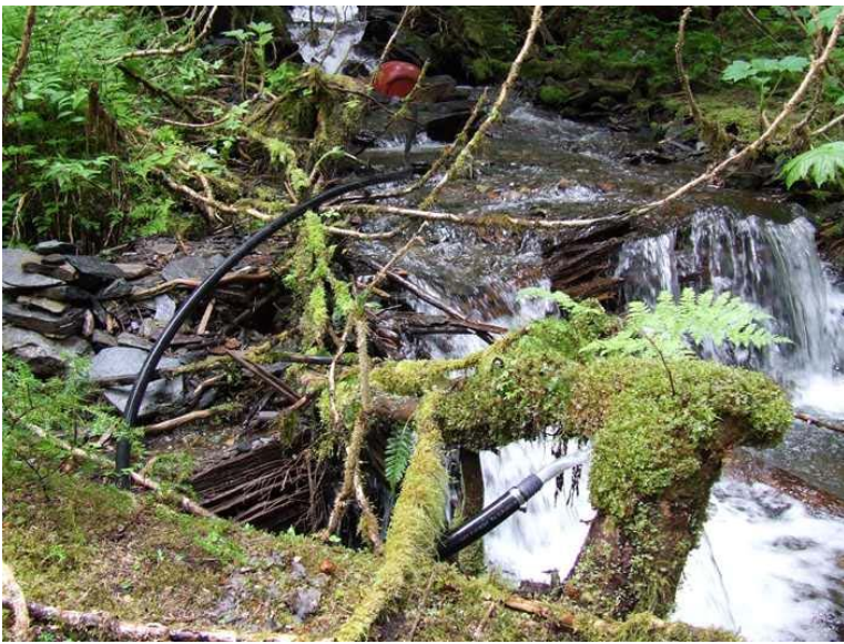
Olive barrel and the first short length of pipe emptying into the creek
