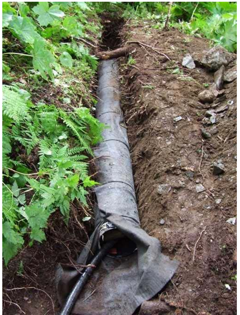
Drain pipe in the trench
