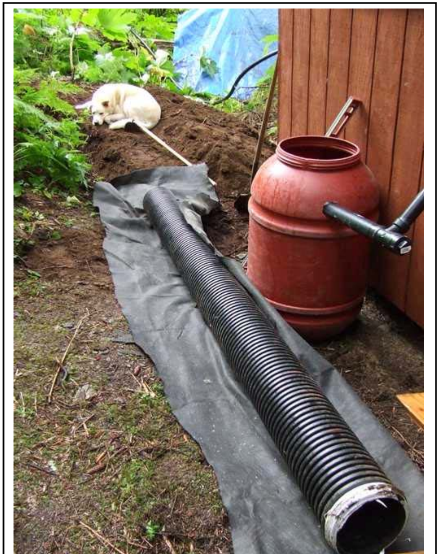
About to wrap felt around the drain pipe
